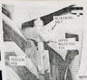
Tension Rod with Self-Locking Nut
