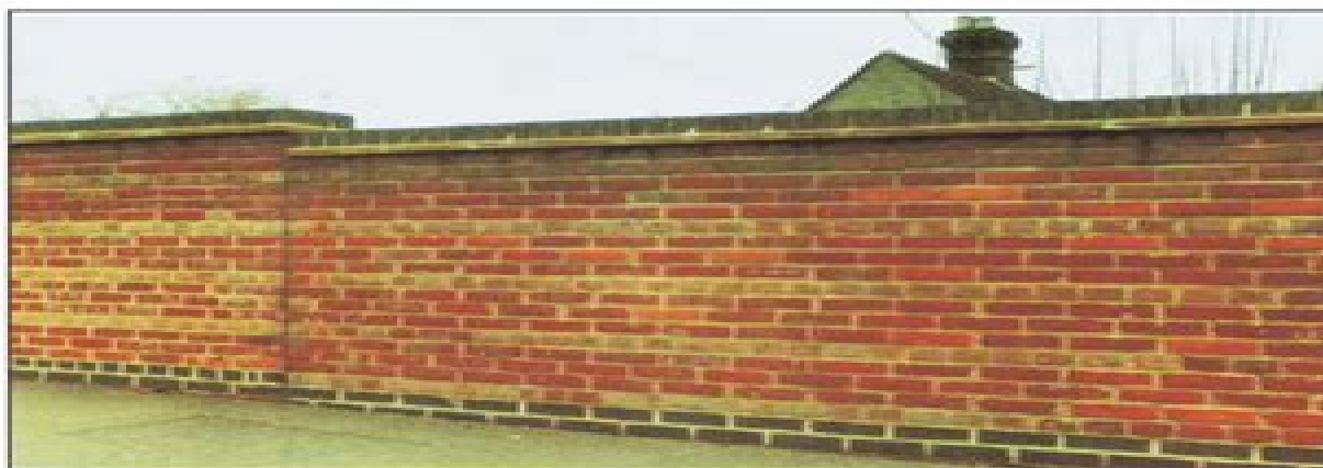
A well constructed wall. The height to thickness ratio makes it safe. Good detailing around the capping and a low level dpc will ensure that it is durable.
