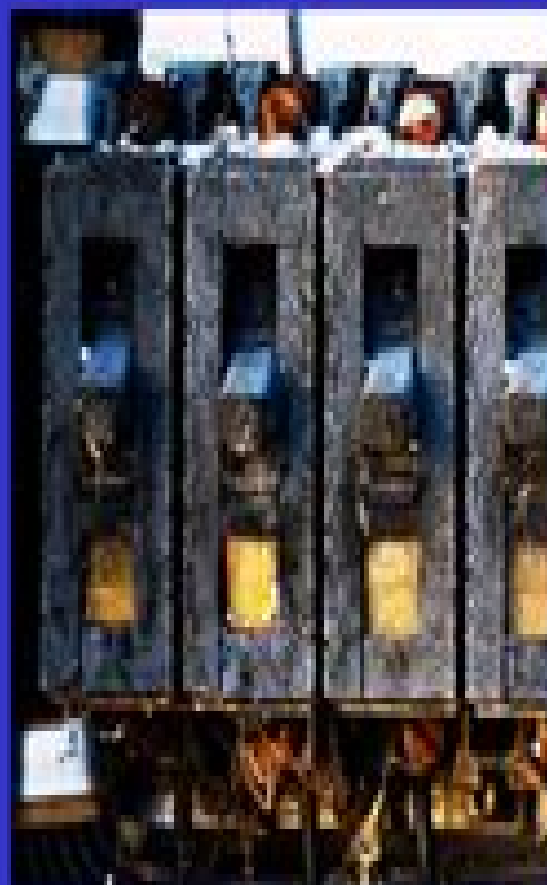
Corrosion or Rust
