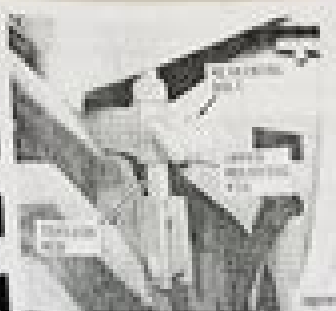
Tension Rod with Self-Locking Nut
